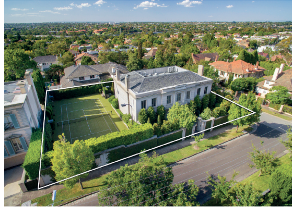
A Nicholas Day Architecture & Marino Construction residence reflecting enduring architecture with a strict adherence to classic proportions.
